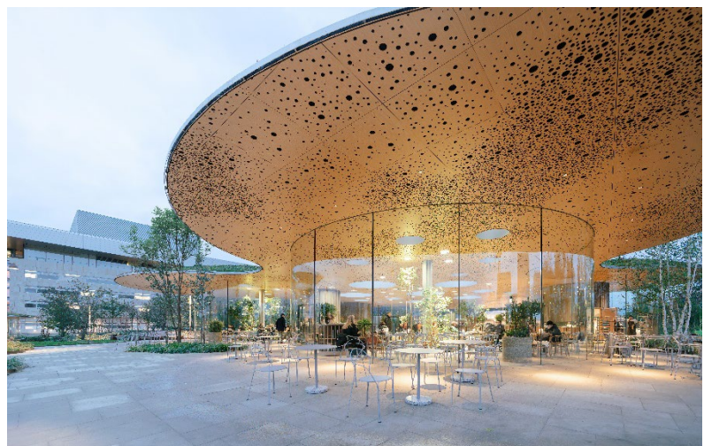
Pavillon Greenhouse, Opera Park, Kopenhagen (Foto: Francisco Tirado)
