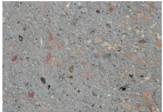
Bild 6 Gestockte Mischabbruch-Recyclingbetonoberfläche Concrete made of recycled aggregate with stacked surface
